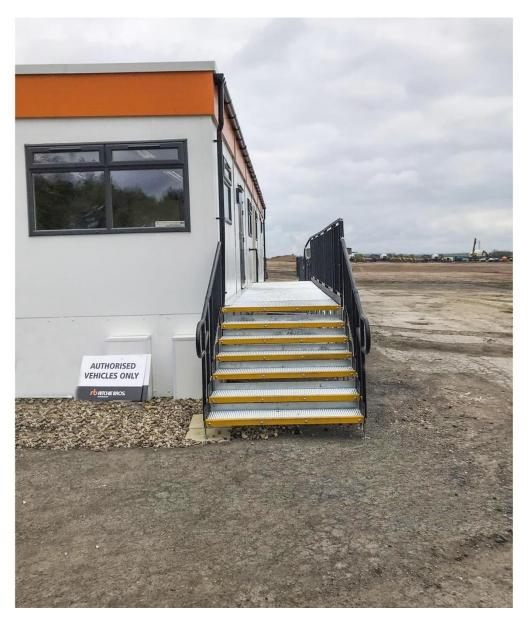
**END RESULT:** Once the groundworks and building were completed, our installation teamed fitted the walkway at the required height with the use of adjustable telescopic legs.
